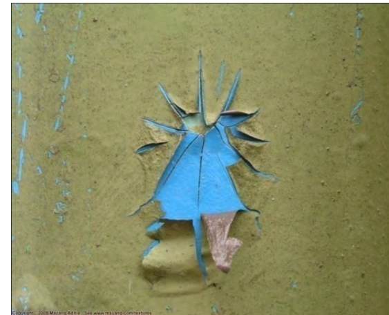
Impact in Metallic Structures Courtesy of SLODIVE
